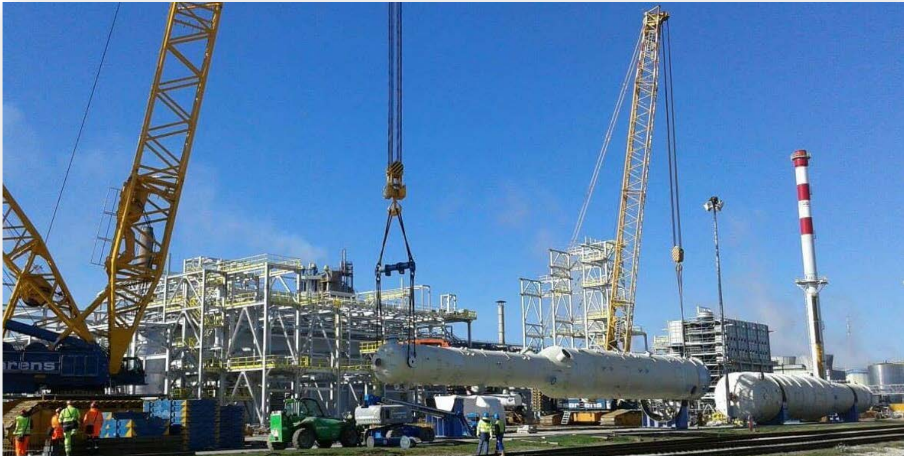
Erection at Sal'A Plant
